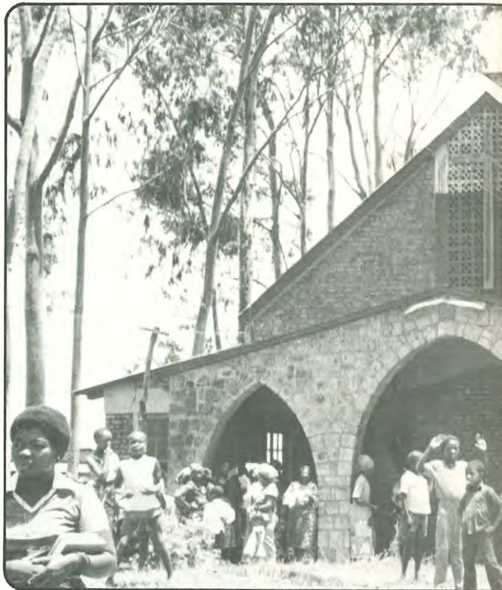
Church at Mbanza Ngungu (above left) Building the 'Peace' at Stanley Pool (top right) M become the headquarters of mission and church work in Bas Zaire.
