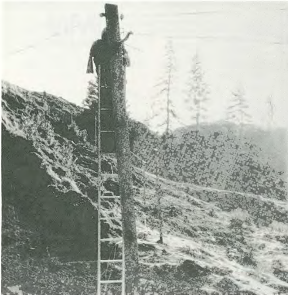
Erecting Poles at Jumla
