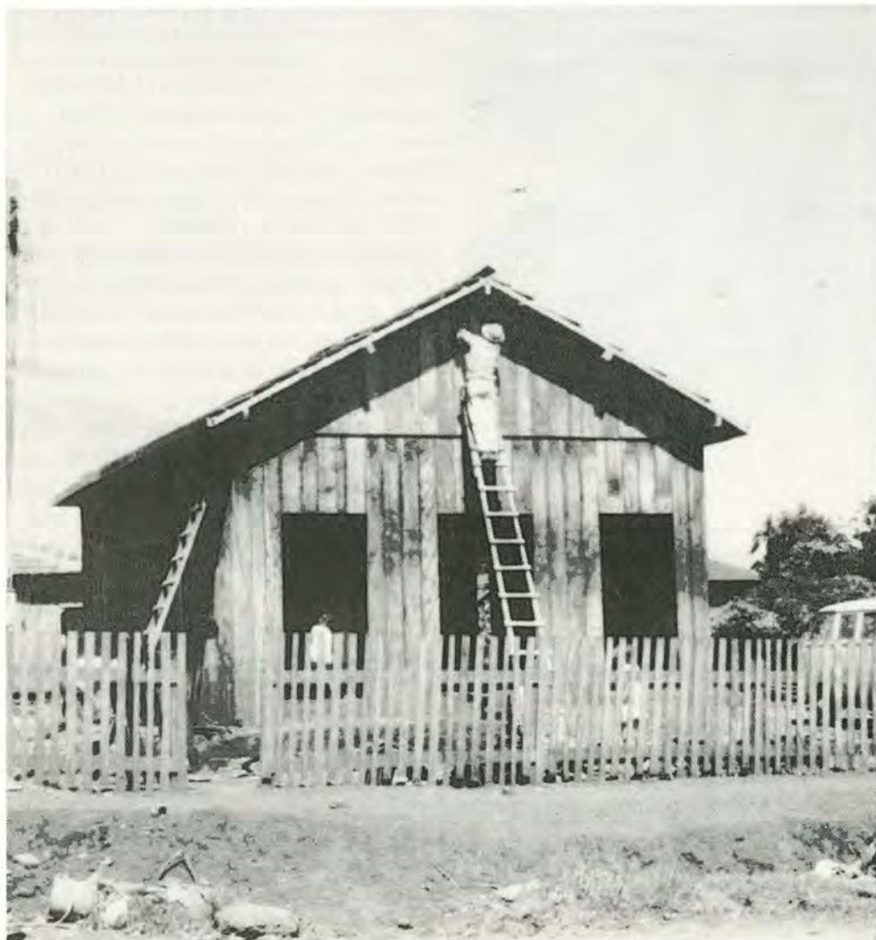
Building the sanctuary at Assis Chateaubriand
