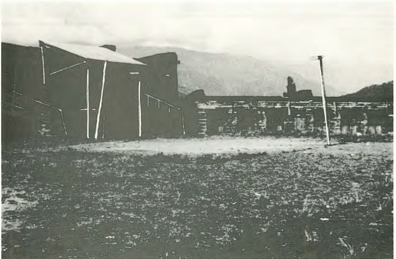
The 'builder's store' school
