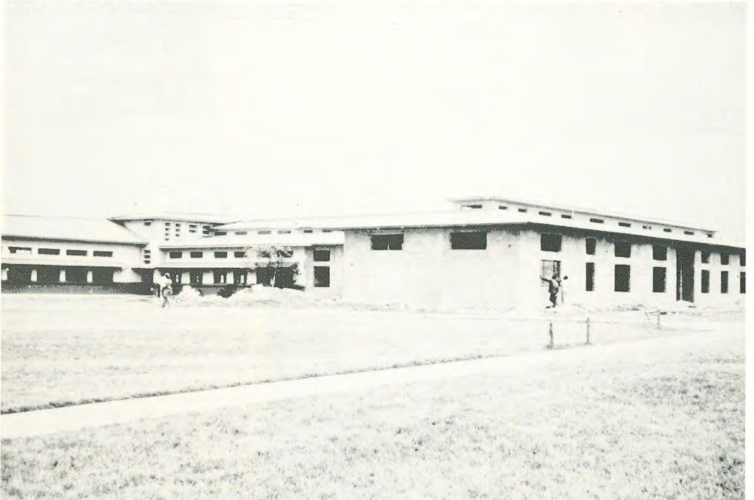
The new theatre and administrative block
