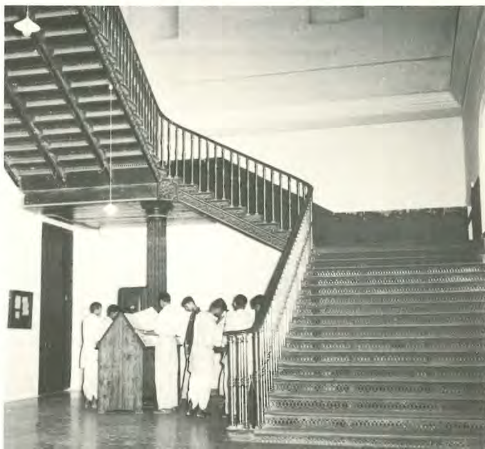
The wrought iron staircase of the main building
