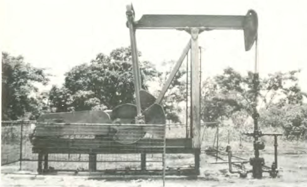
Oil well near Point Fortin
