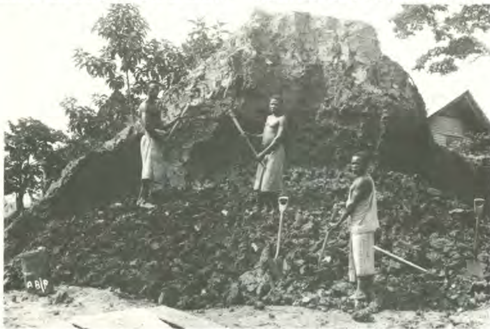
Digging clay for bricks from white ant hill
