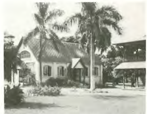
Calabar Chapel, now used by the High School
