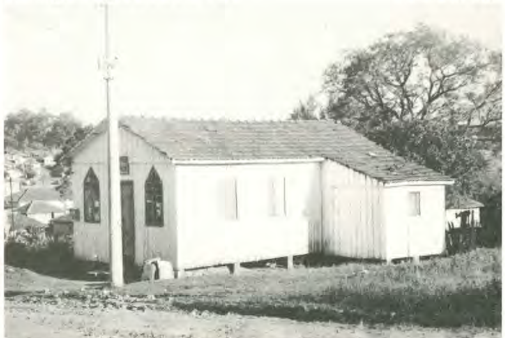
The 'temporary' church building at Santo Antonio da Platina
