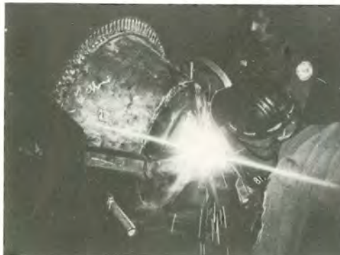
Welding at Butwal
