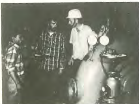
Power house, Butwal
