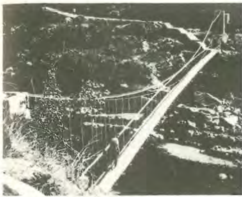
Bridge built by United Mission to Nepal
