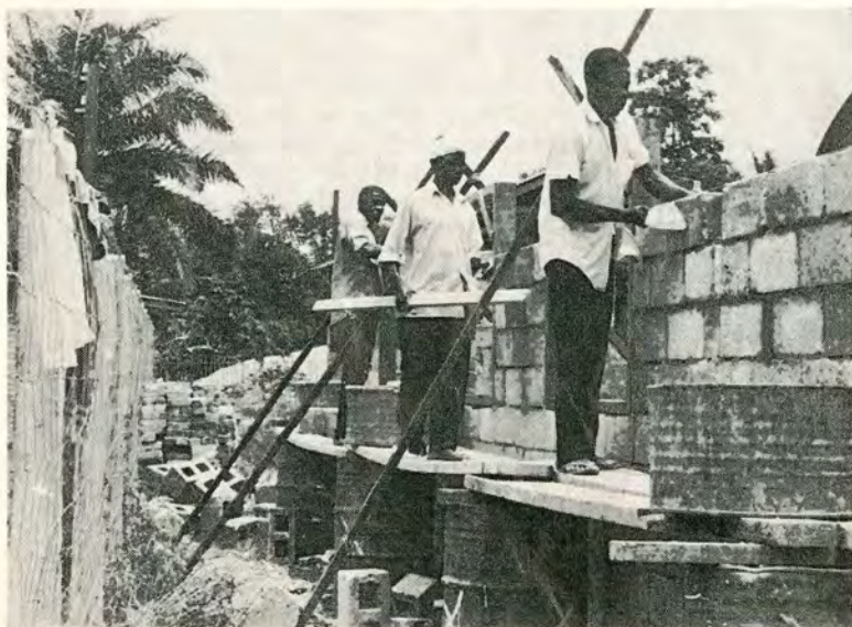
Building the hospital chapel at Bolobo.
